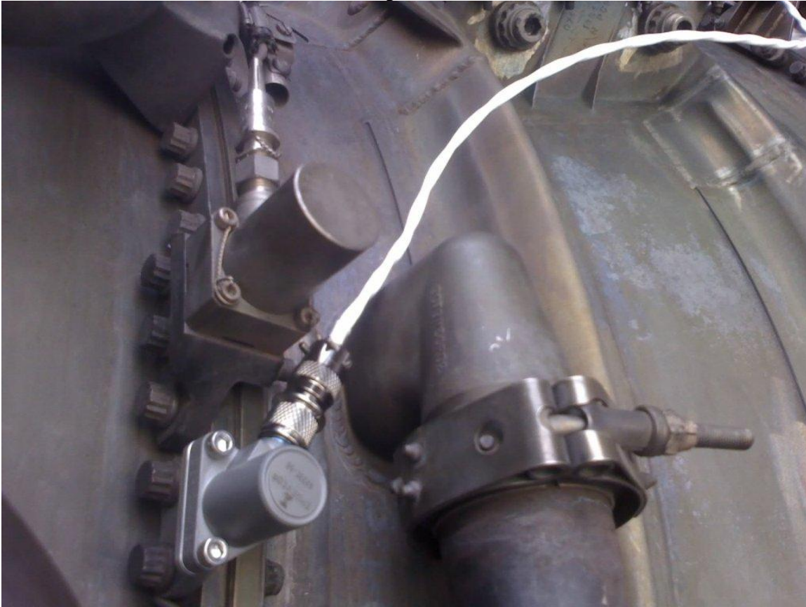
Figure 3. Sensor installed on the mount with high temperature cable attached and routed toward top of engine.
